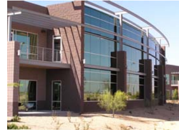
Even new buildings should have a PCA performed
