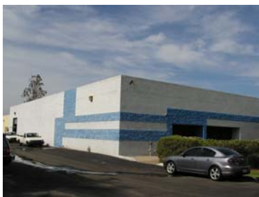
Many industrial sites with septic tank systems require an APP
